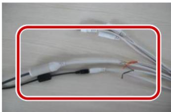
2. Protect the connected cables using insulating tapes.
